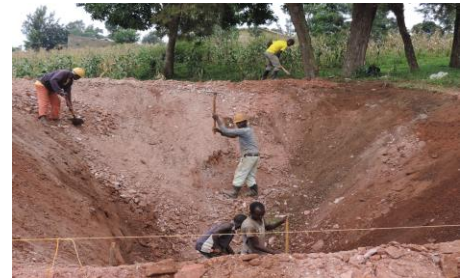
Preparation of dams for smart irrigation.
